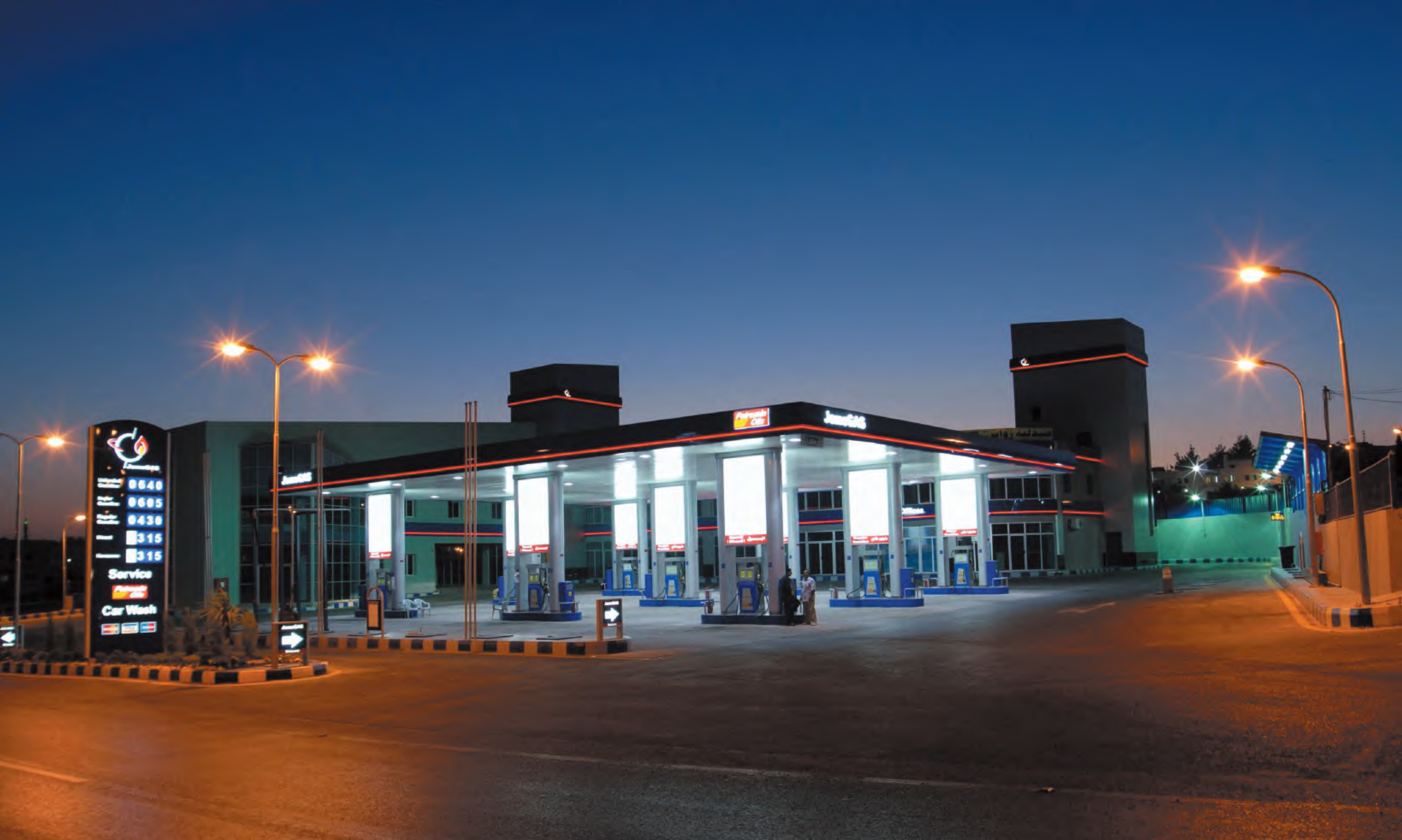
Manaseer Gas Station - (Total of 80 Gas Stations)
